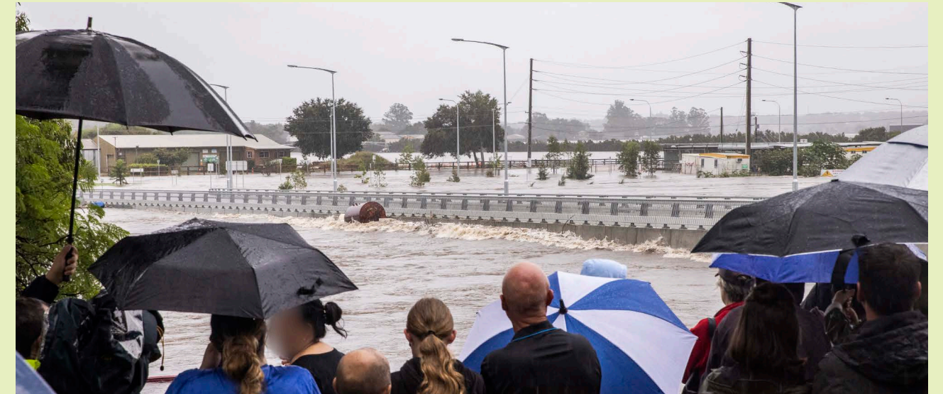
Image: New Windsor Bridge, major flood event (2022).
