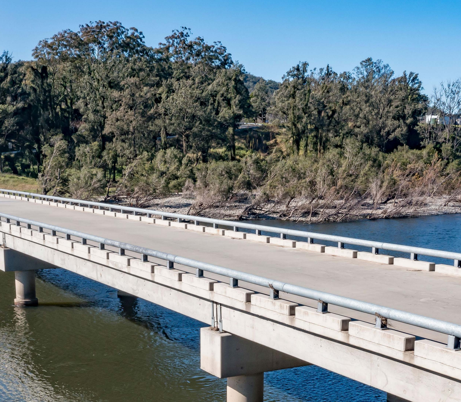
Image: Turners Flat Replacement Bridge, Northern NSW (2022).
