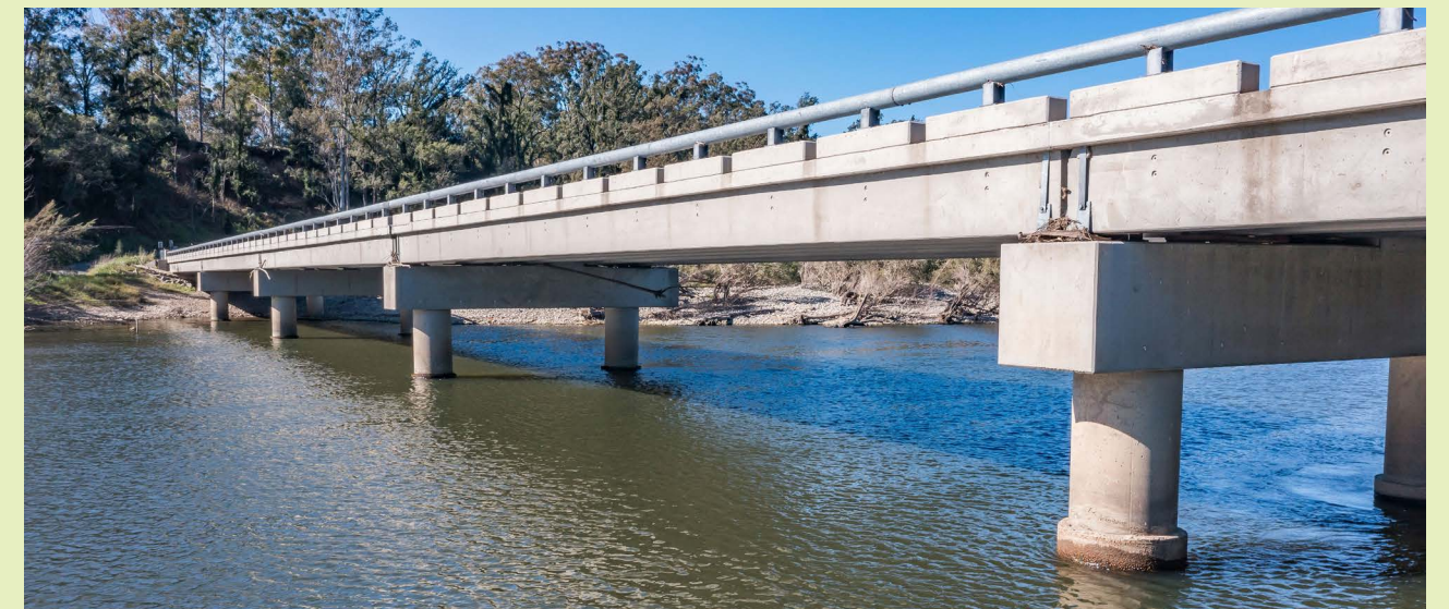
Image: Turners Flat Replacement Bridge, Northern NSW (2022).
