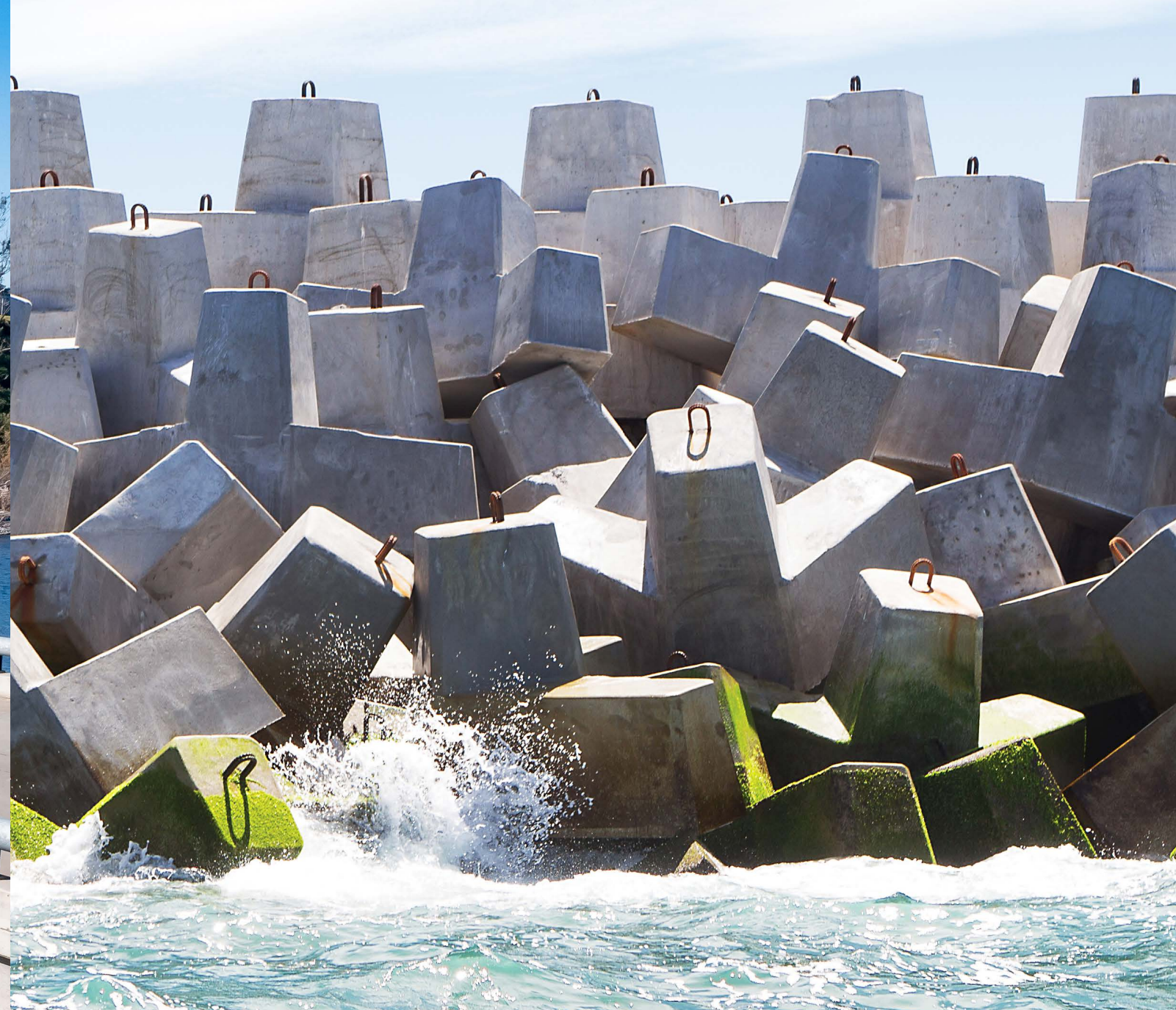
Image: Coffs Harbour Eastern Breakwall Project (2014).
